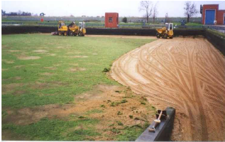
Plate 2.1 - Cleaning a full-scale slow sand filter at Walton, Thames Water
